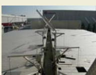
Industrial SBR of Barcelona ECOPARC to leachate treatment
